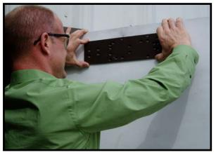
**Step Three:** Align holes in the mounting plate with the exisiting mounting holes in the door. Flip plate if closer being replaced is mounted in parallel arm application.
